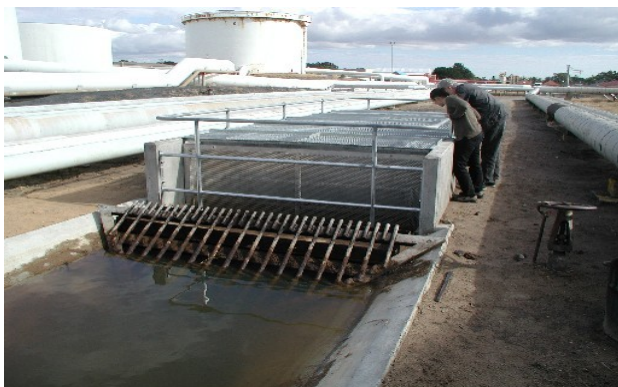
EGOWS Installation at Kurnell Oil Refinery, Sydney
